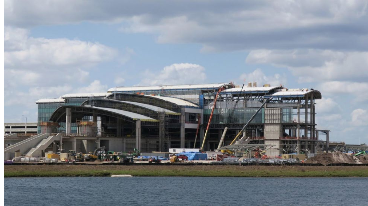
Orlando International Terminal C during construction
