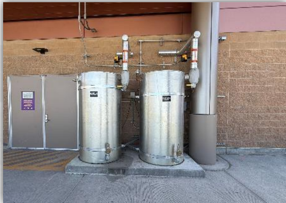
Liquid Oil Waste Extraction & Grease Interception System (5,000 Gallon Tanks in Ramp)
