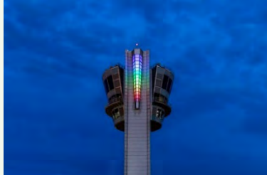
(Courtesy of Philadelphia International Airport)
