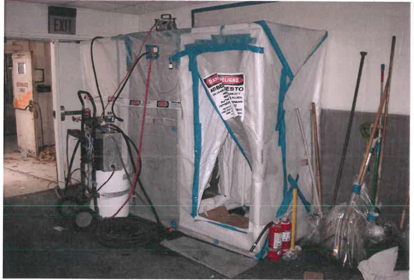
Photo 4 View of Decontamination Chamber for Asbestos Abatement
