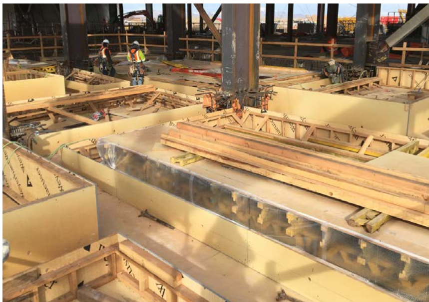
Mid-Concourse Tunnel Concrete Lid forms
