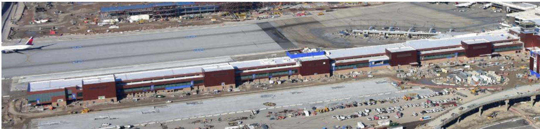
SCW Building Exterior – Areas 'A' through 'H', looking north
