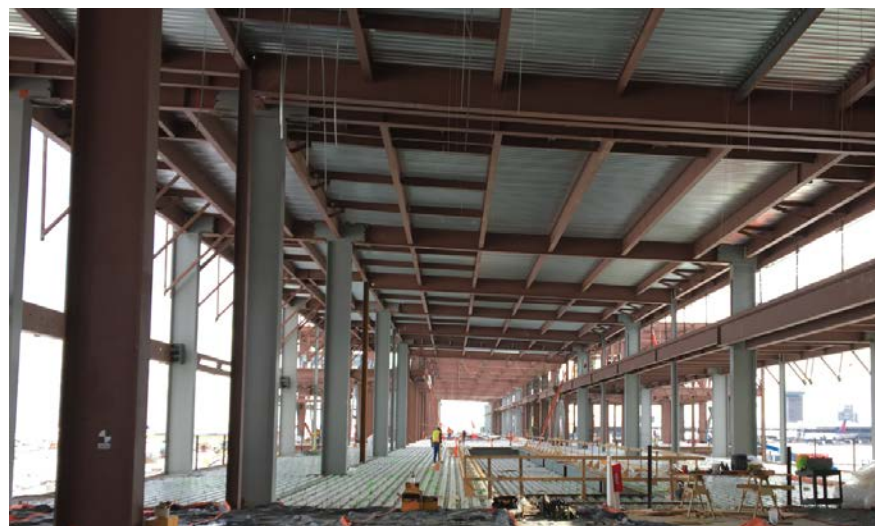
North Concourse Sector 'B' Level 2 looking east
