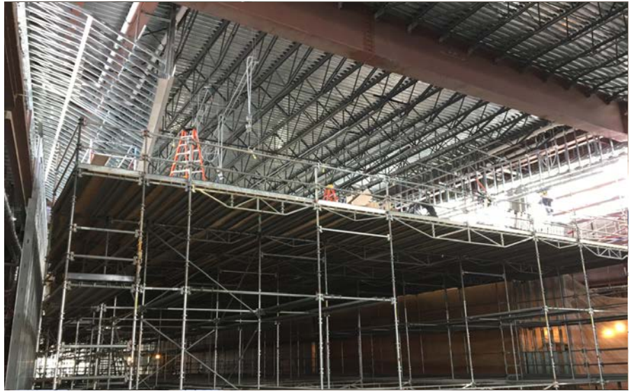
Terminal Canyon High-Bat Scaffolding Section 3
