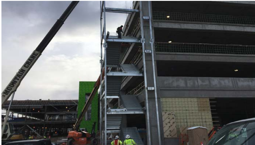
Parking Garage NW Stair installation
