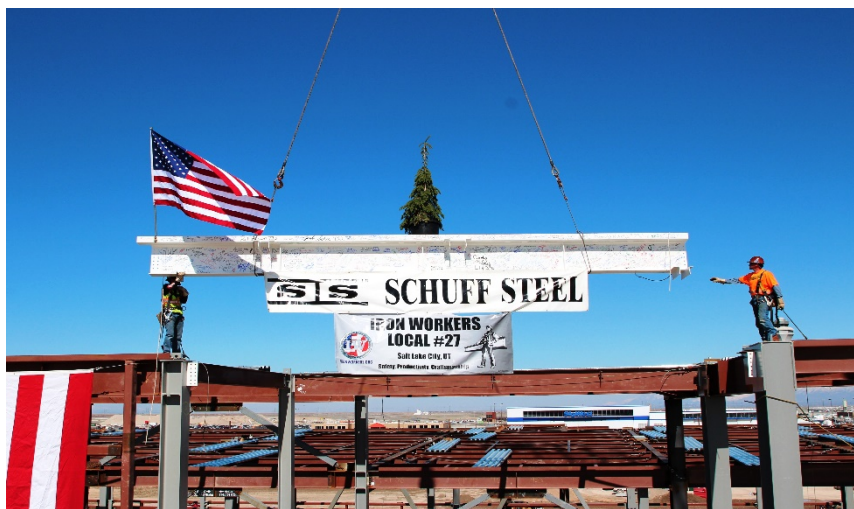
North Concourse Steel Erection Topping-out
