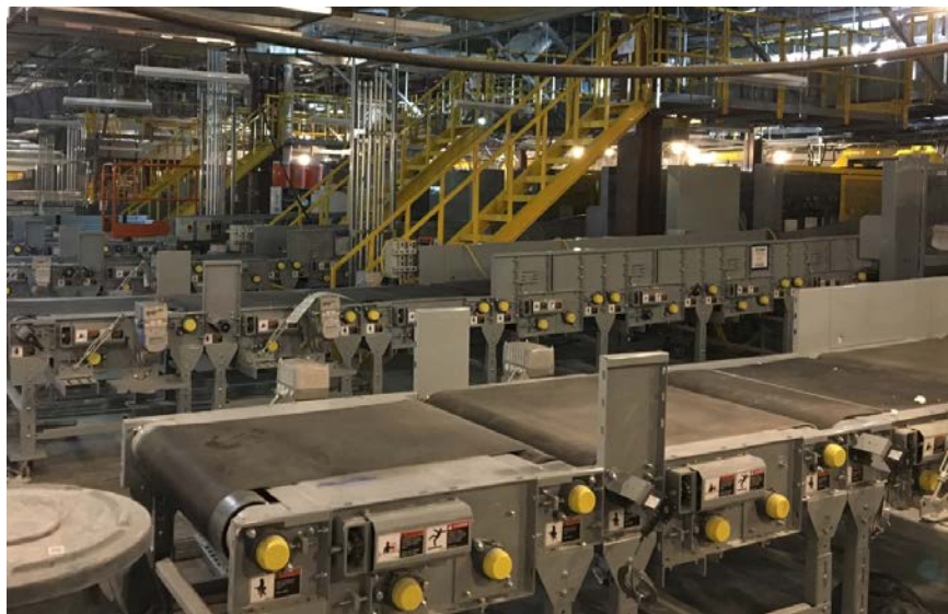
CBIS Terminal Area 'A'
