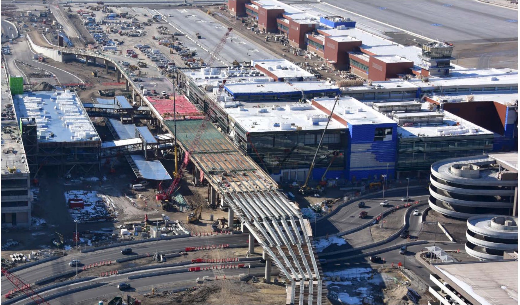
Terminal, Gateway, and Elevated Roadway, looking west
