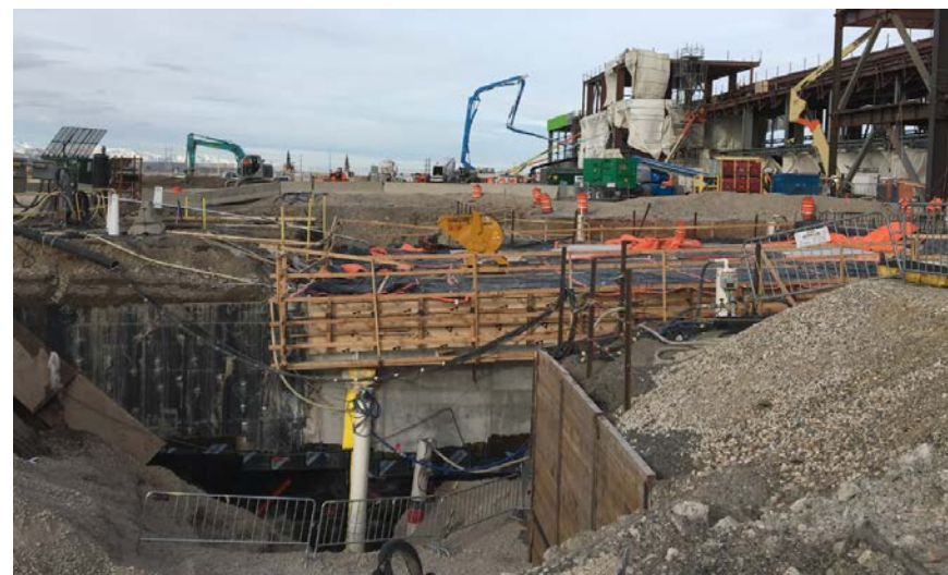
Mid-Concourse Tunnel Sector 'CN'
