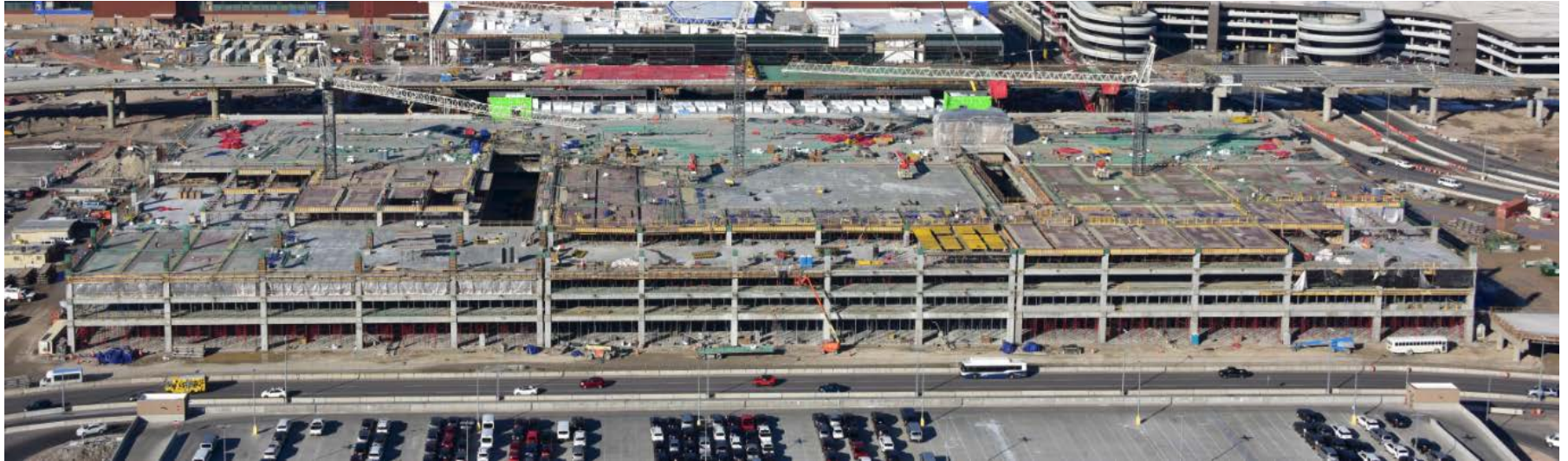
Parking Garage looking north
