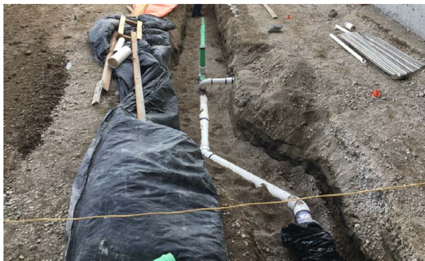
North Concourse Sector 'D' Shallow Underground Piping
