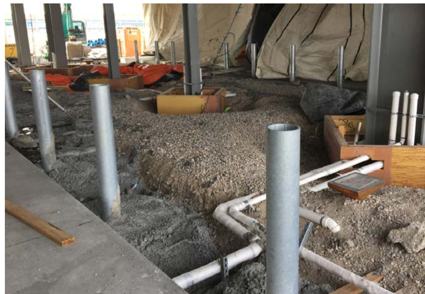
North Concourse Sector 'B' Breezeway
