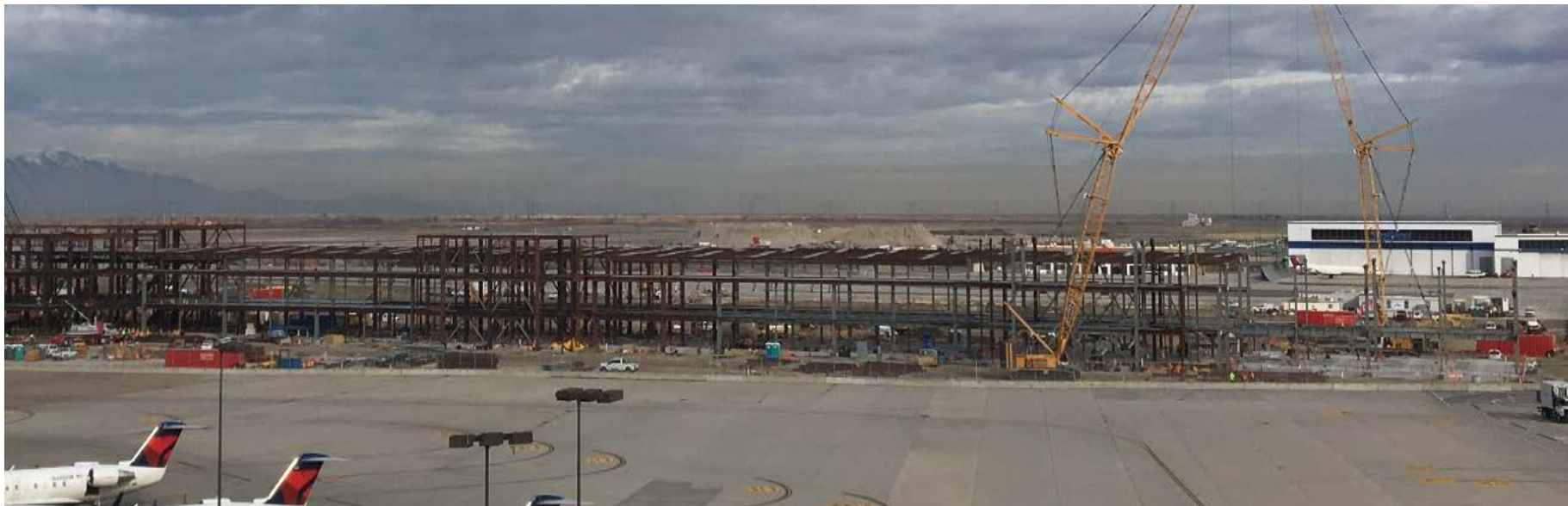
North Concourse Steel erection, Sectors 'CN' through 'F' (east end), looking north
