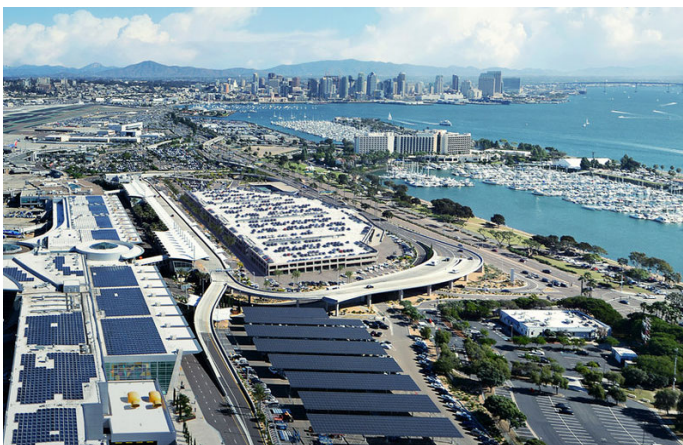
SDIA Terminal 2 Parking Plaza; Photo: Swinerton, Inc.
