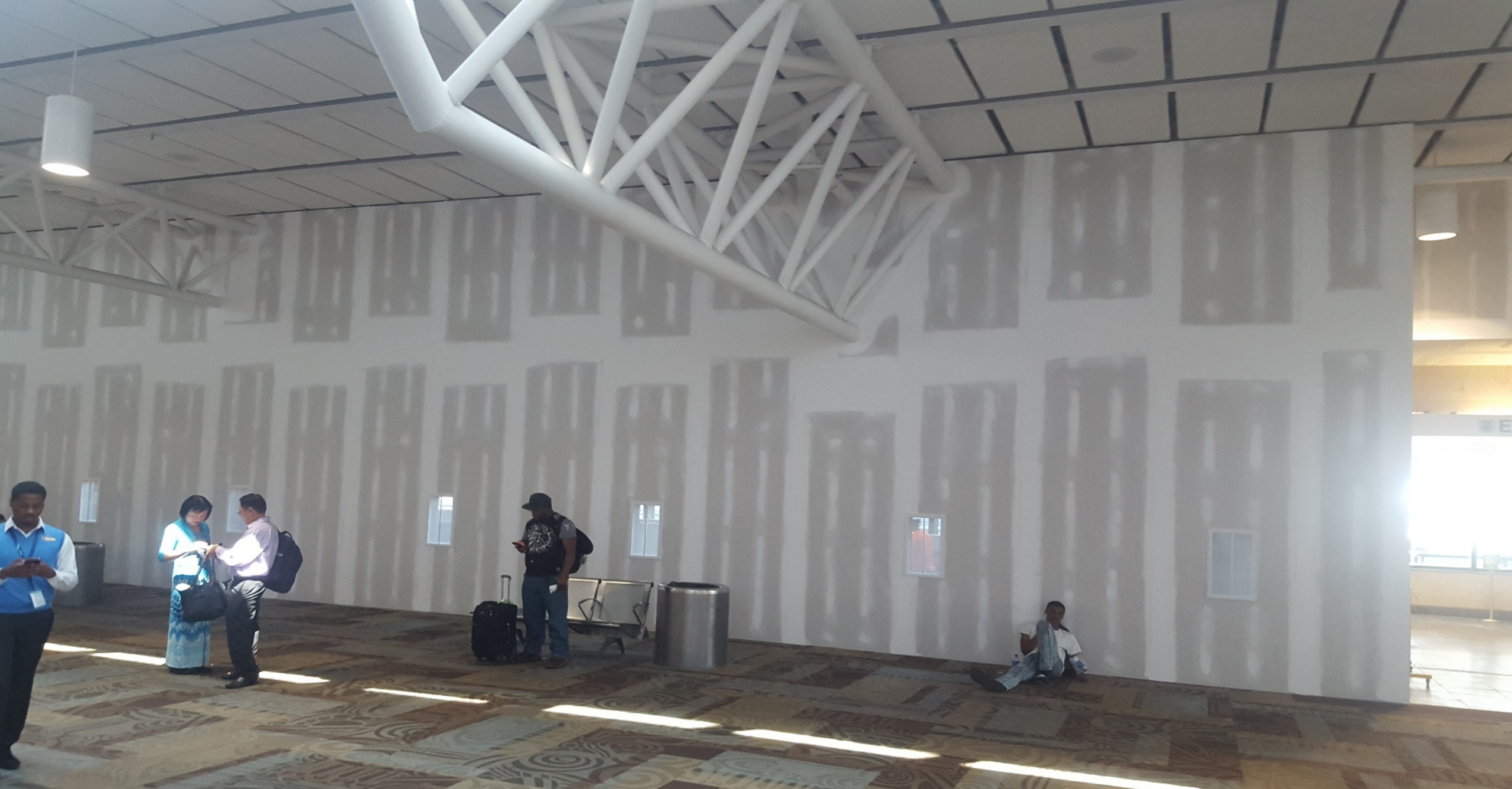
Concourse D Expansion
