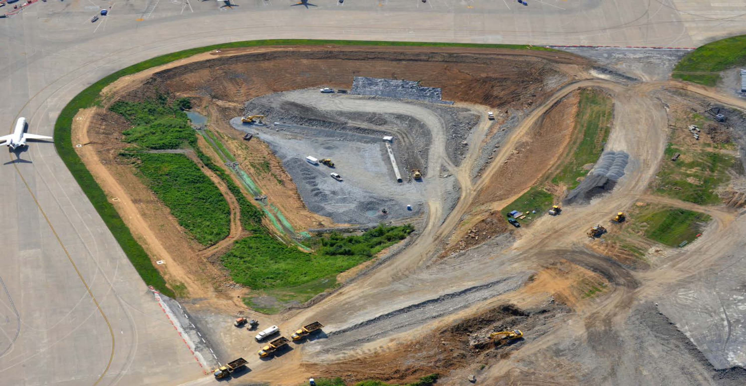
Apron Expansion – July 2018
