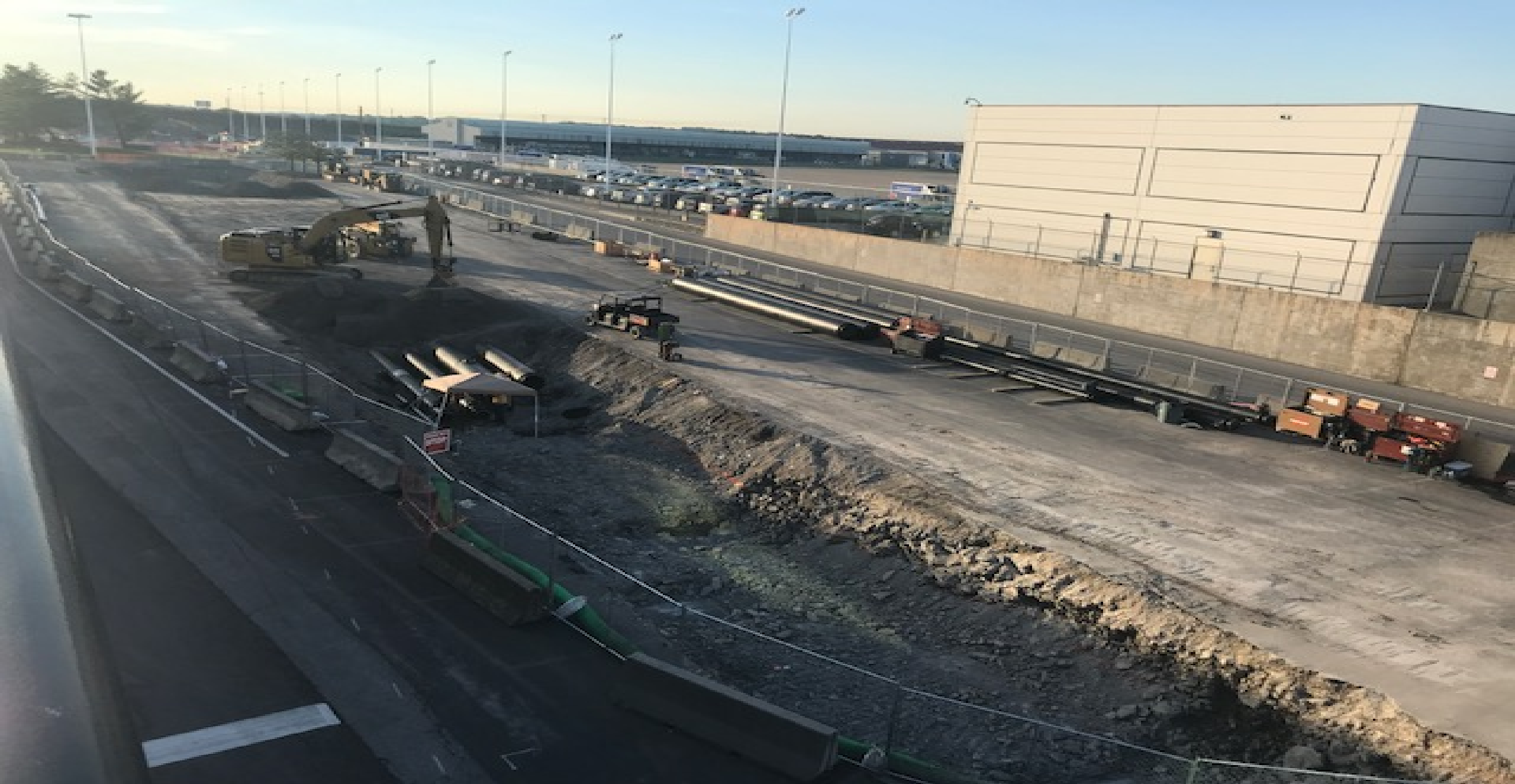
Concourse D Expansion
