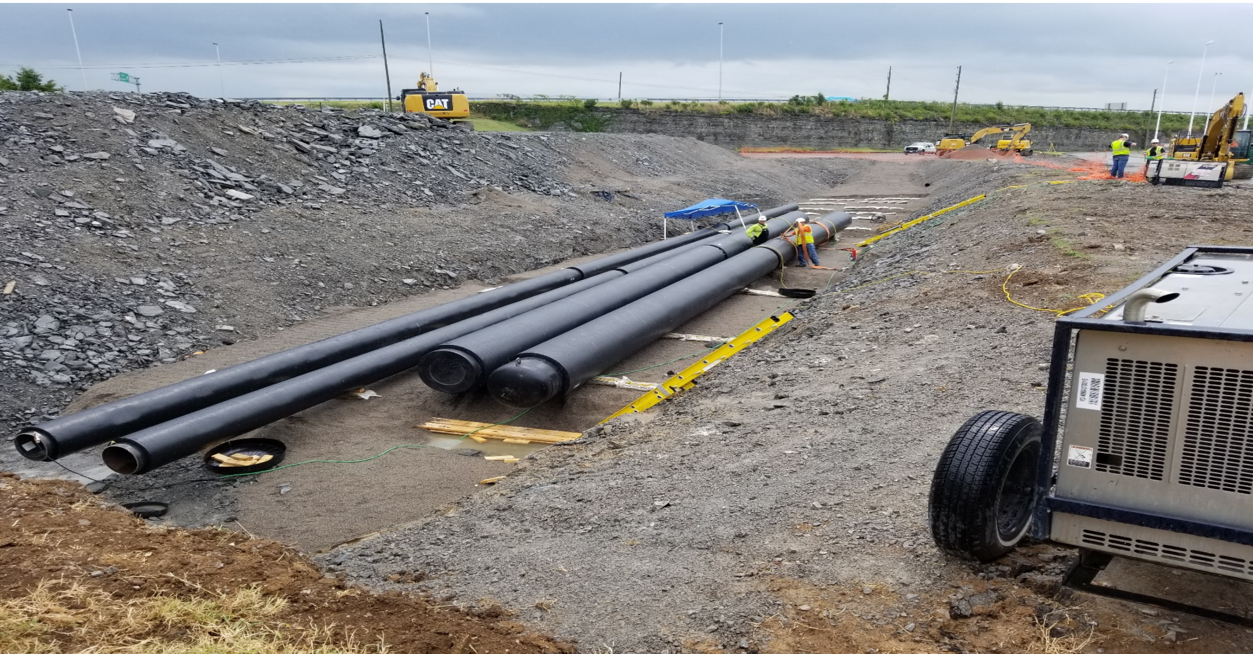
Concourse D Expansion
