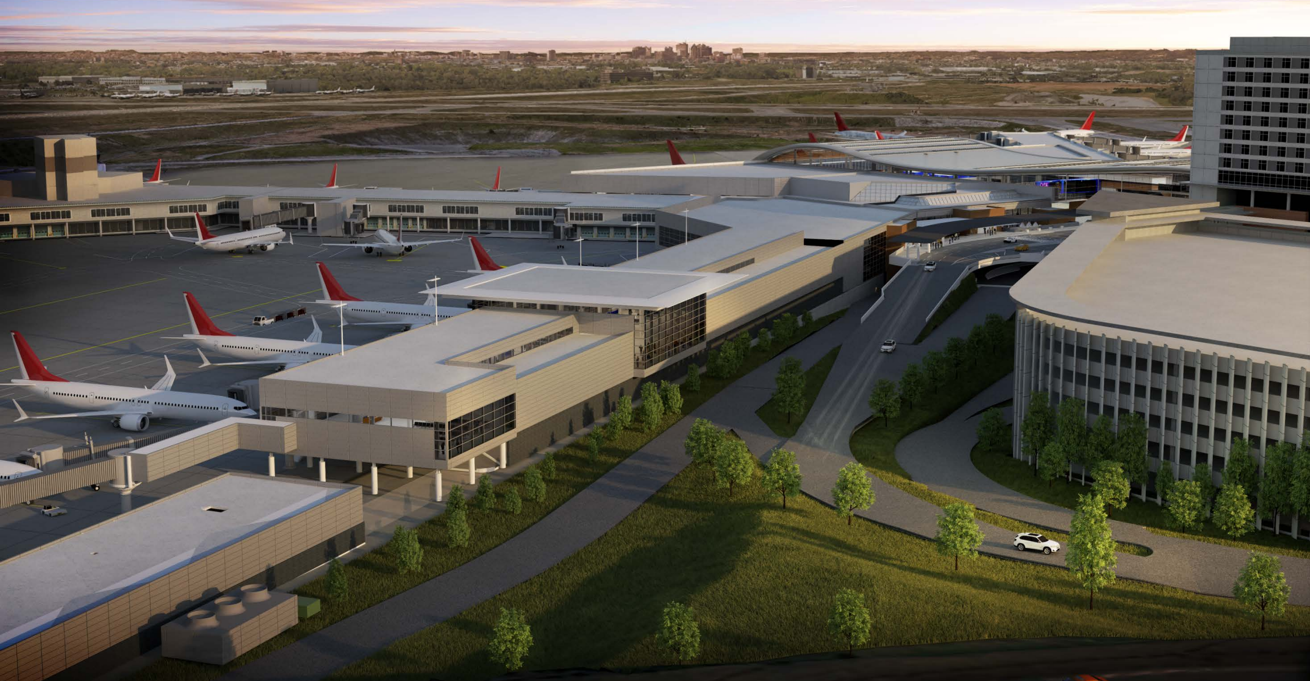
Concourse D Expansion
